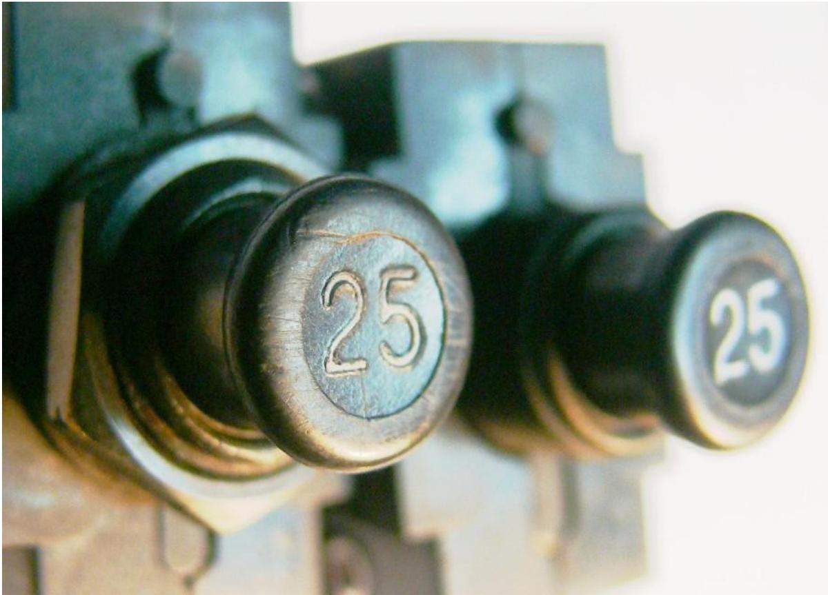
Fig. 9. Buttons of C829 circuit breakers (left – from SP-LPC, right – a new one)
